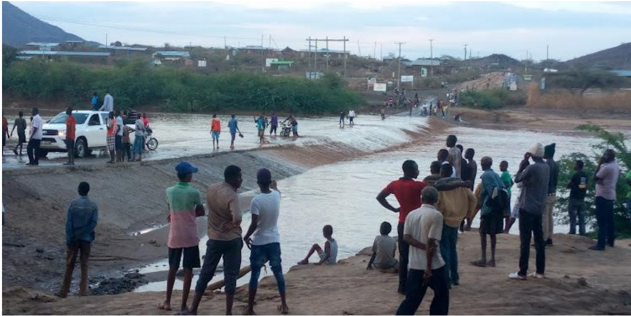
Figure 2: A flooded drift on a road in Turkana
